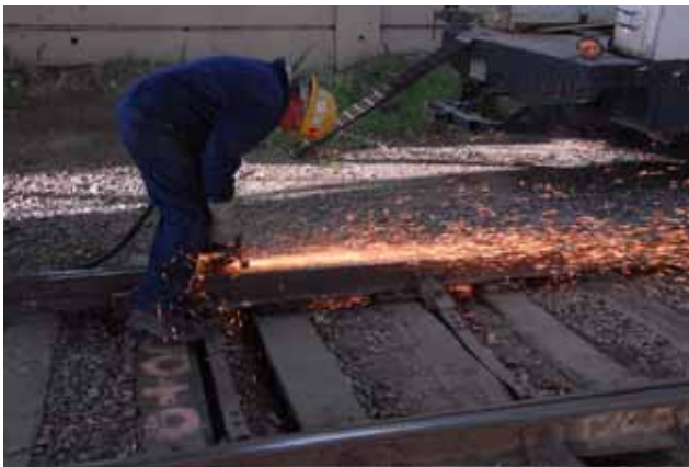
Greg Copeland Repairing Switch Point
