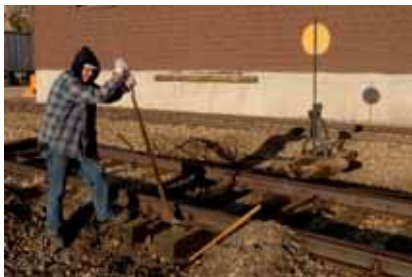
Don Hulse Removing Switch at Federal Center
