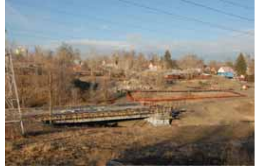
RTD West Corridor Light Rail Bridge Just West of Perry Under Construction on Jan. 24, 2009
